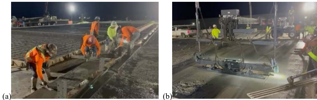
Figure 1. Manual (a) and laser (b) screeding examples for slab-on-grade construction
