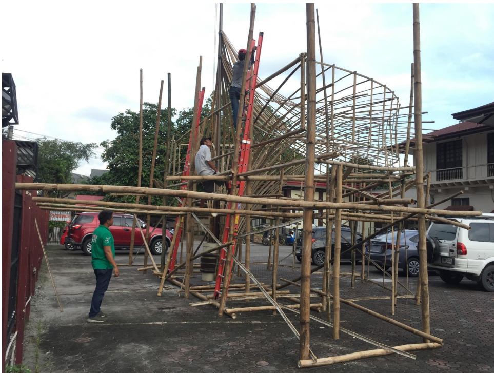
Figure 2: Craftsmen working on the bamboo formwork.
