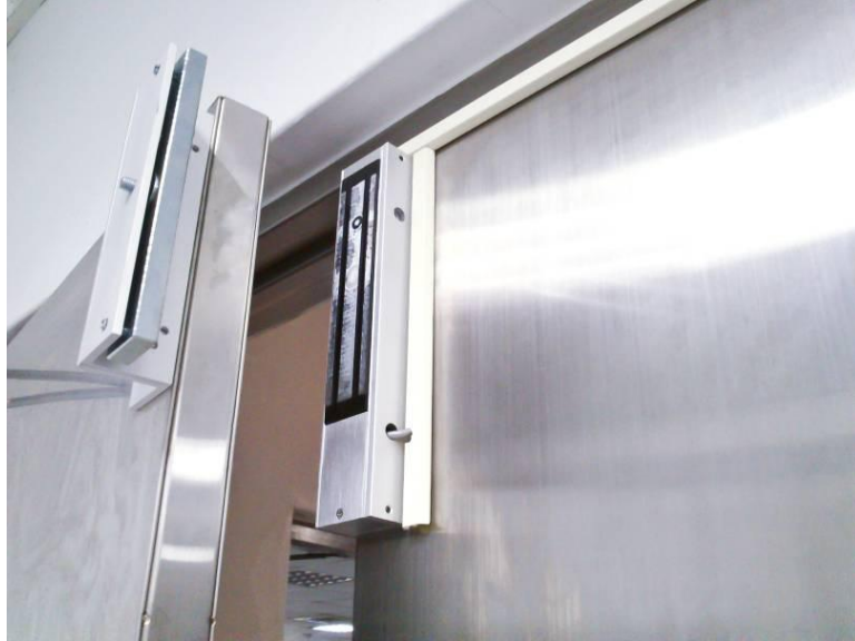
Figure 4.1 Magnetic lock
