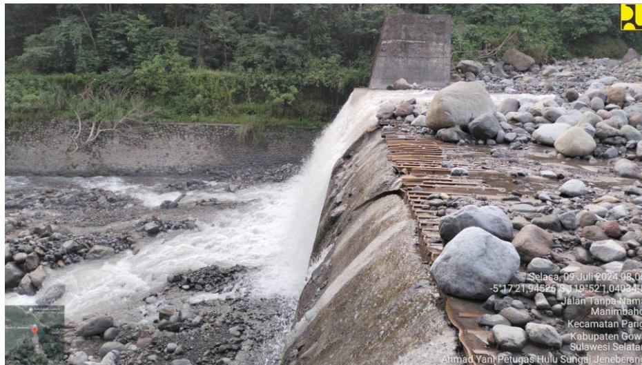
Figure 2: Sabo Dam 7.1 Jeneberang River
