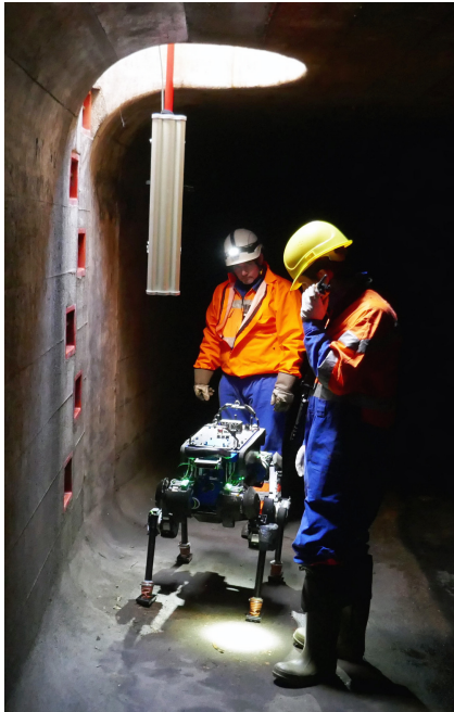
(a) ANYmal setup in the sewer
