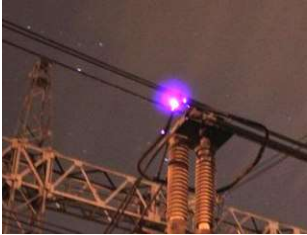
Fig. 1. Corona effect in a transmission line [10]
