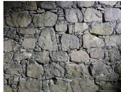
FIGURE 1. Bedding Mortar for The Large Stones
